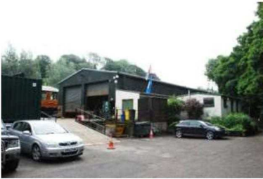
Current Repair Shed
