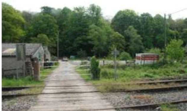
The current User Worked Level Crossing
