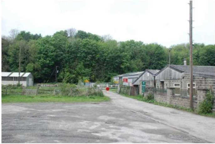
Level crossing with the car park on the left. View looking west.
