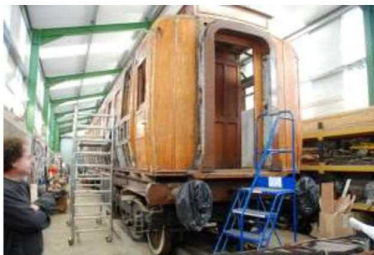
Internal view of the current LNER Carriage shop
