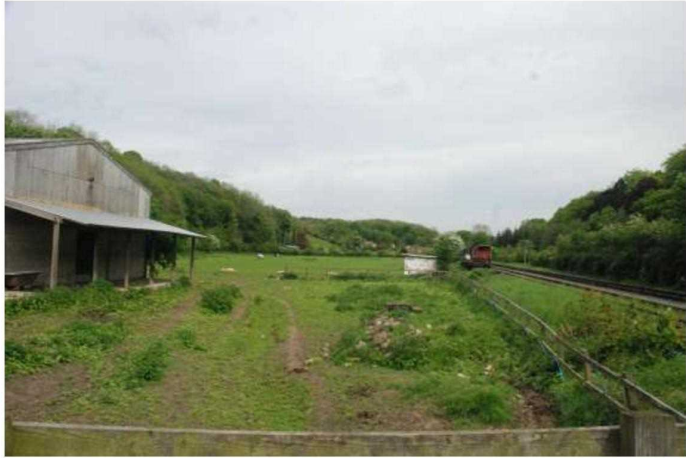
Entrance to the site, view looking north
