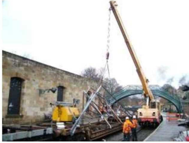
Construction of the new overall station roof utilising materials brought to site by rail
